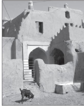
Fig. 8: Renovation of Garme's small inn (photo: authors)
