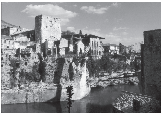
Fig. 2: Destroyed Old Bridge in Mostar, 1996 (photo: author's archive)
