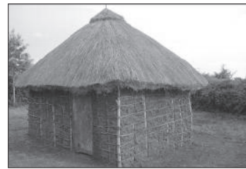
Fig. 4: Completed house before finishing touches are made on the walls, which are continuously smeared with red mud and cow dung for protection from pests and aesthetic purposes. Originally the doors were made from woven reeds and tough animal hides, but currently iron sheets are used for security purposes (Ojoo, 2009).
