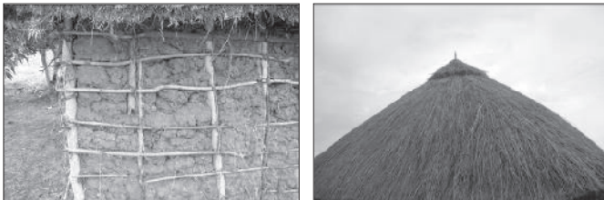
Fig. 3: Wall and roof of a grass-thatched Luo traditional house (Ojoo, 2009).
