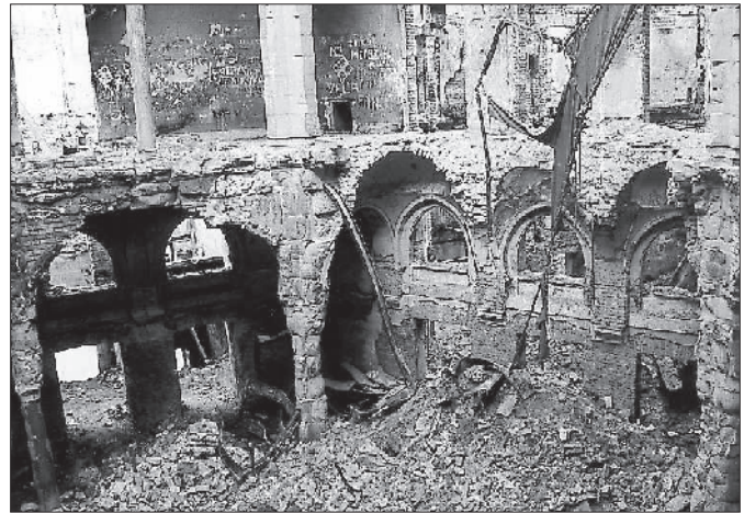
Fig. 1: Interior of the National and University Library of Bosnia-Herzegovina, Sarajevo, 1996 (photo: author's archive)
