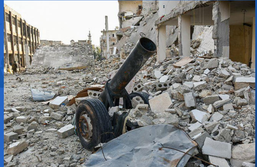
8.2) Destroyed City of Aleppo, Syria,
