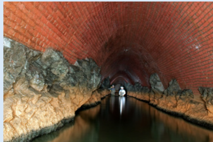
● What does mining have to do with the Freiberg district hospital? Students learned how the underground mine water in the mining town of Freiberg is used to provide sustainable ventilation and geothermal energy to the hospital today.
